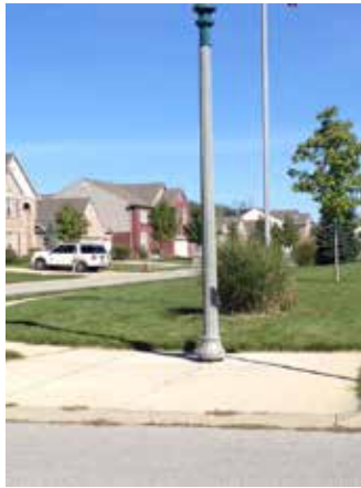
Street Light Encroaching Bayfield Dr. and Bayhill Cir.
