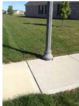
Street Light Encroaching Port Dr.
