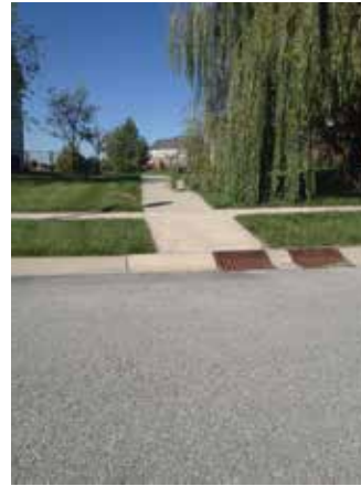
No Ramp/Curb Inlet Barrier Crestview Tr.
