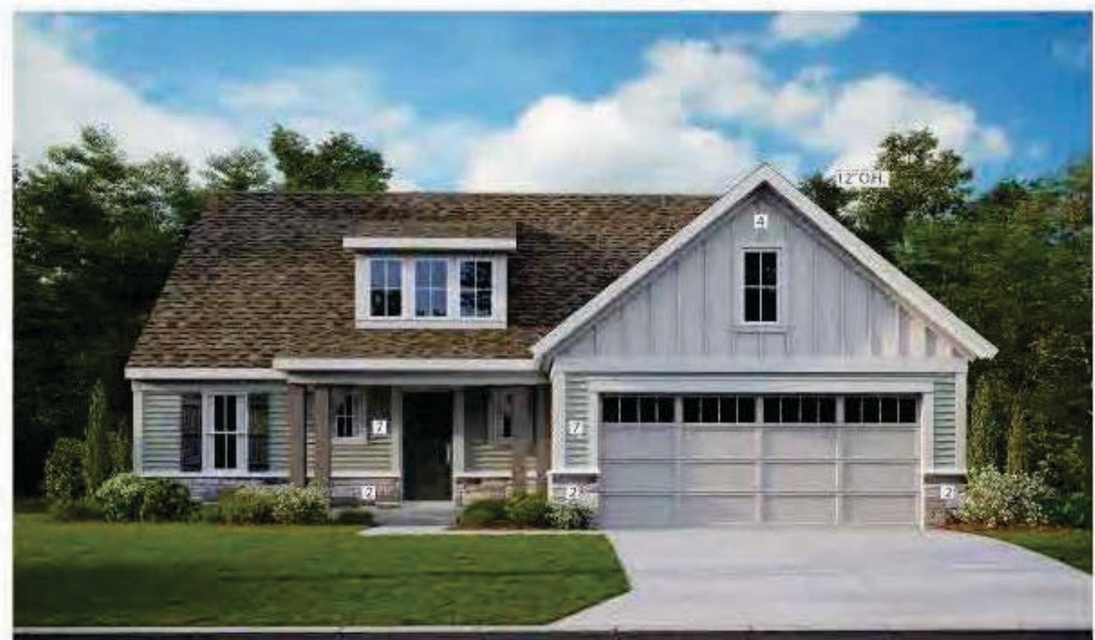
KEATON - MODERN FARMHOUSE W/ STONE STONE (2) = 26% HARDI-PANEL (4) = 33% VINYL HORIZONTAL SIDING (7) = 41% TOTAL MASONRY = 59%
