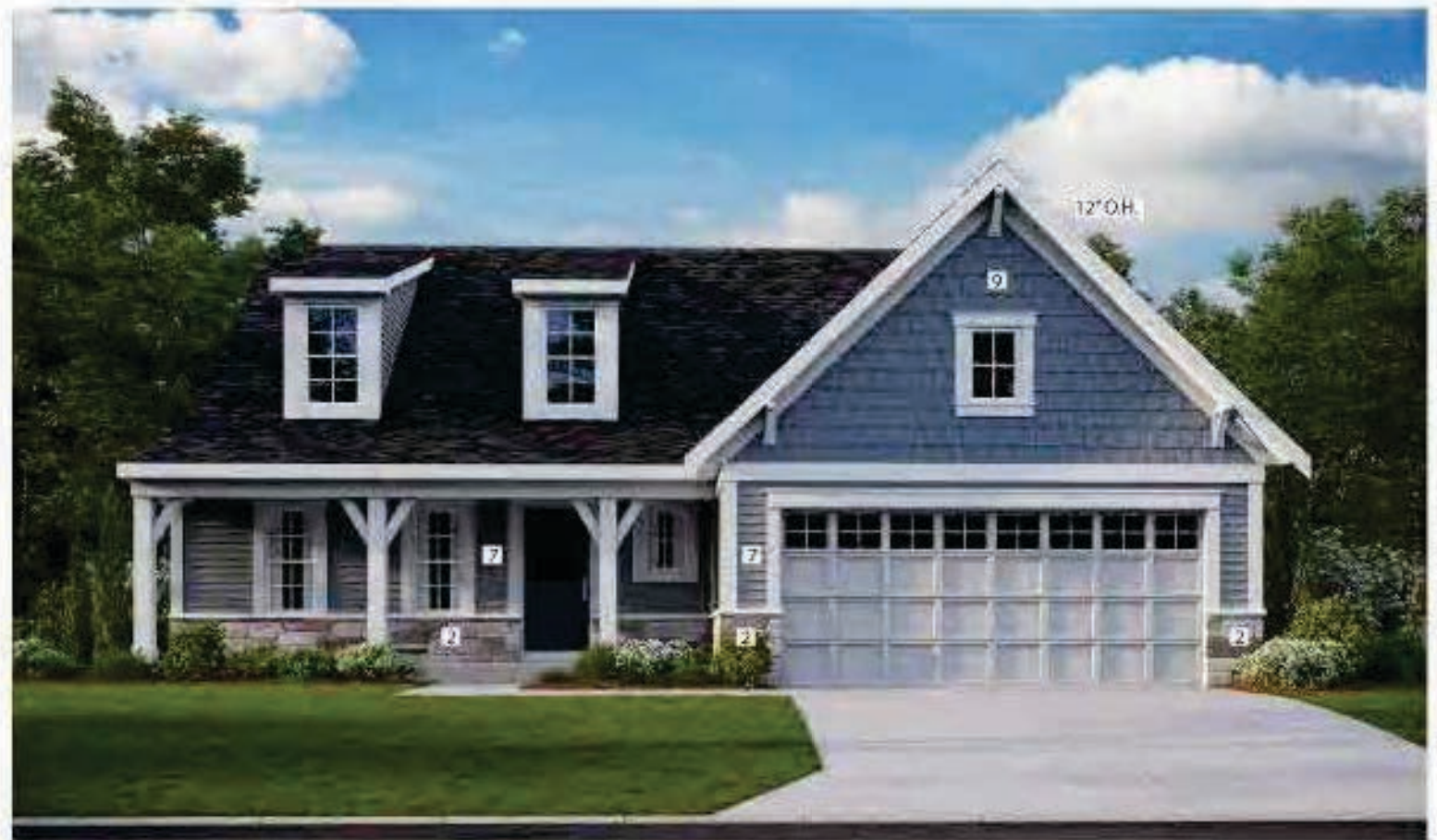
KEATON - AMERICAN FARMHOUSE W/ STONE STONE (2) = 27% VINYL, HORIZONTAL SIDING (7) = 41% HARDI-PANEL SHAKE SIDING (9) = 29% TOTAL MASONRY = 56%
