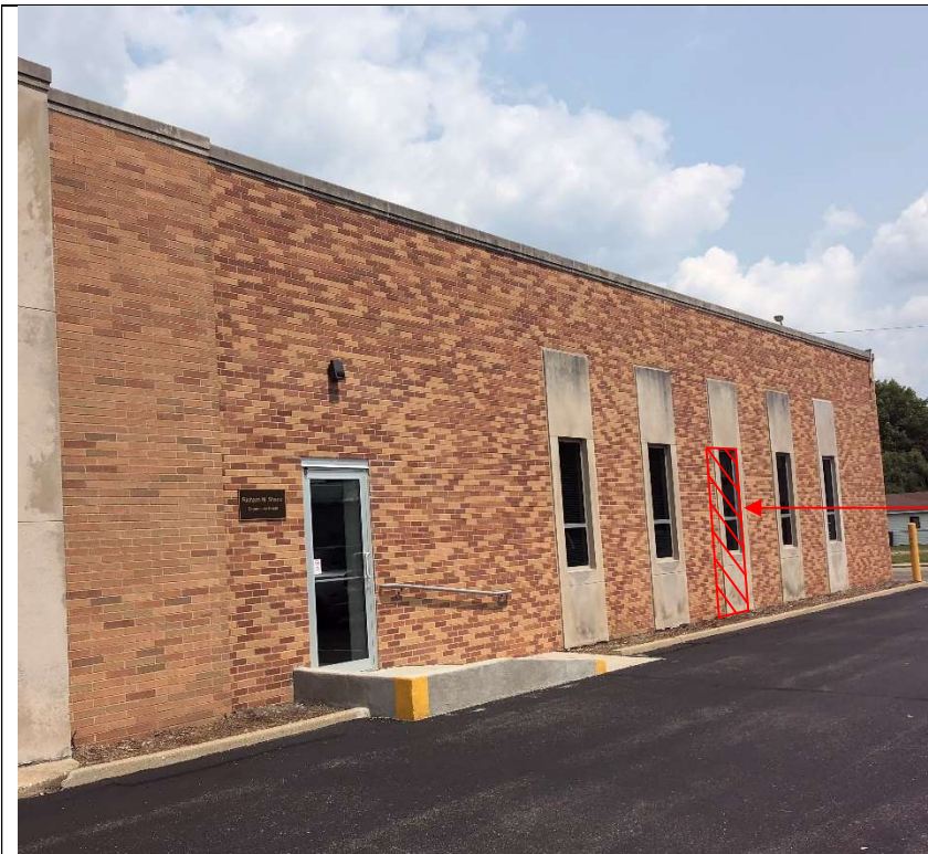
Photograph No. 1 Description: View of south exterior façade with entrance door into Community Center
