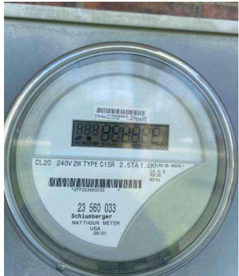
UTILITY COMPANY: Ninestar Connect
