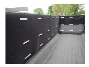
Hypernet 200 is approximately 3/16" thick diamond pattern heavy polypropylene drainage fabric. This material will never rust and is tough and UV resistant to last many years. It can easily be replaced if needed by removing the aluminum strips and installing new pieces in a minimal amount of time and with little labor.
