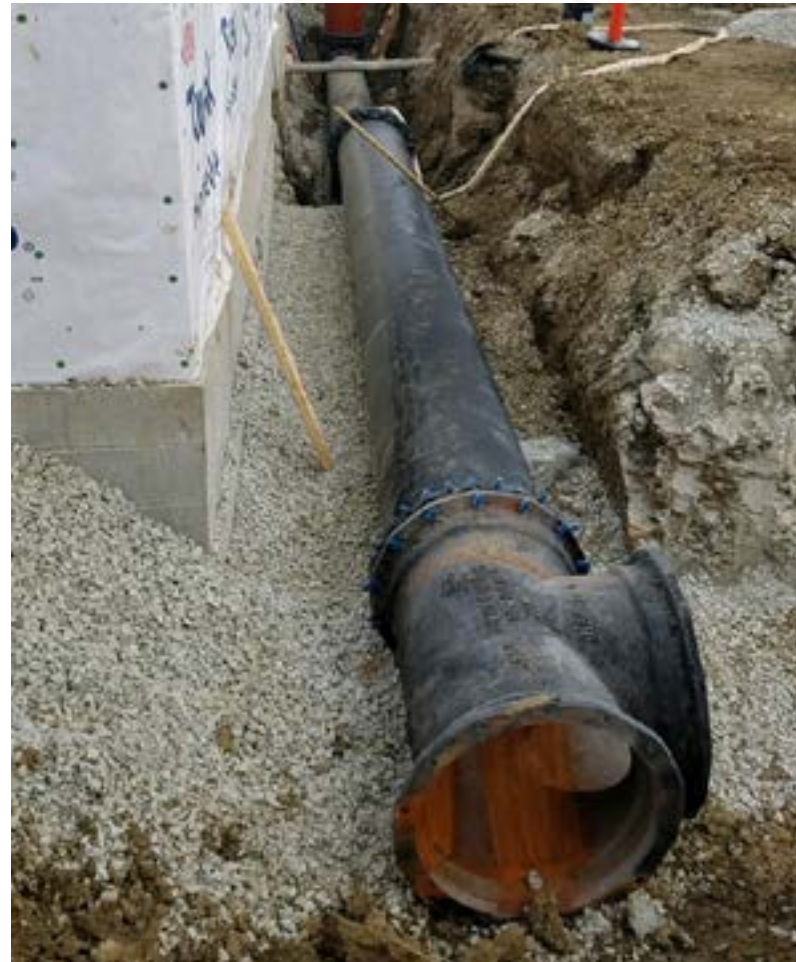
The Wastewater Treatment Plant expansion will double the current capacity.
