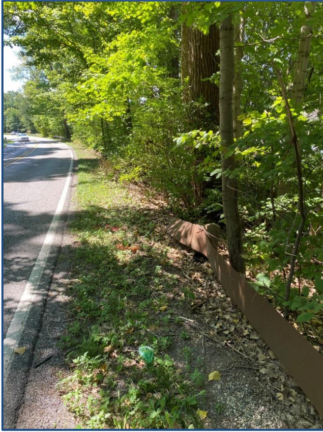
Figure 1: Face of guardrail at the north end of the guardrail limits. Large trees located within the clear-zone.
