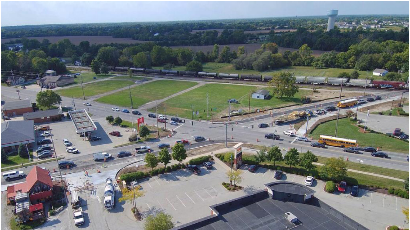
Right turn lanes made at the intersection of CR 600W and Broadway have helped provide a smoother flow of traffic.
